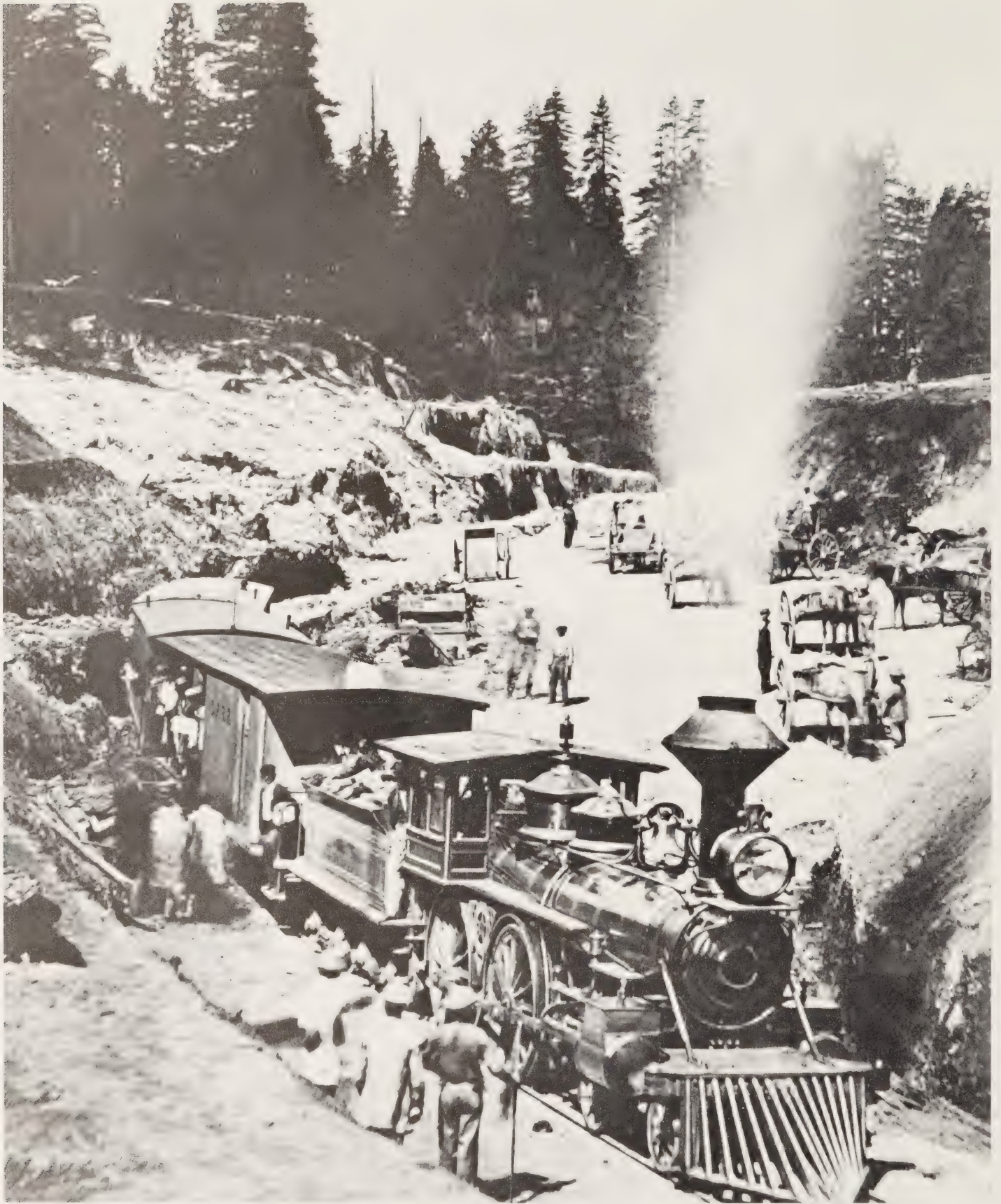
Central Pacific Work Train in the Sierra Mountains During 1865 When the Railroad Grade was Being Cut Above Auburn. Chinese Working with Picks and Shovels, One-Horse Dump Carts and Black Powder Carved a Right-of-Way Through Solid Granite.
